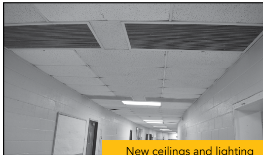
New ceilings and lighting
