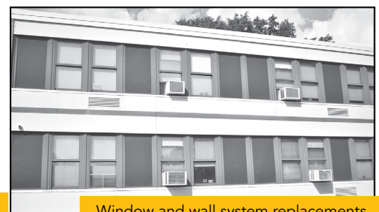
Window and wall system replacements
