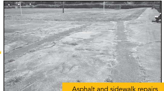
Asphalt and sidewalk repairs
